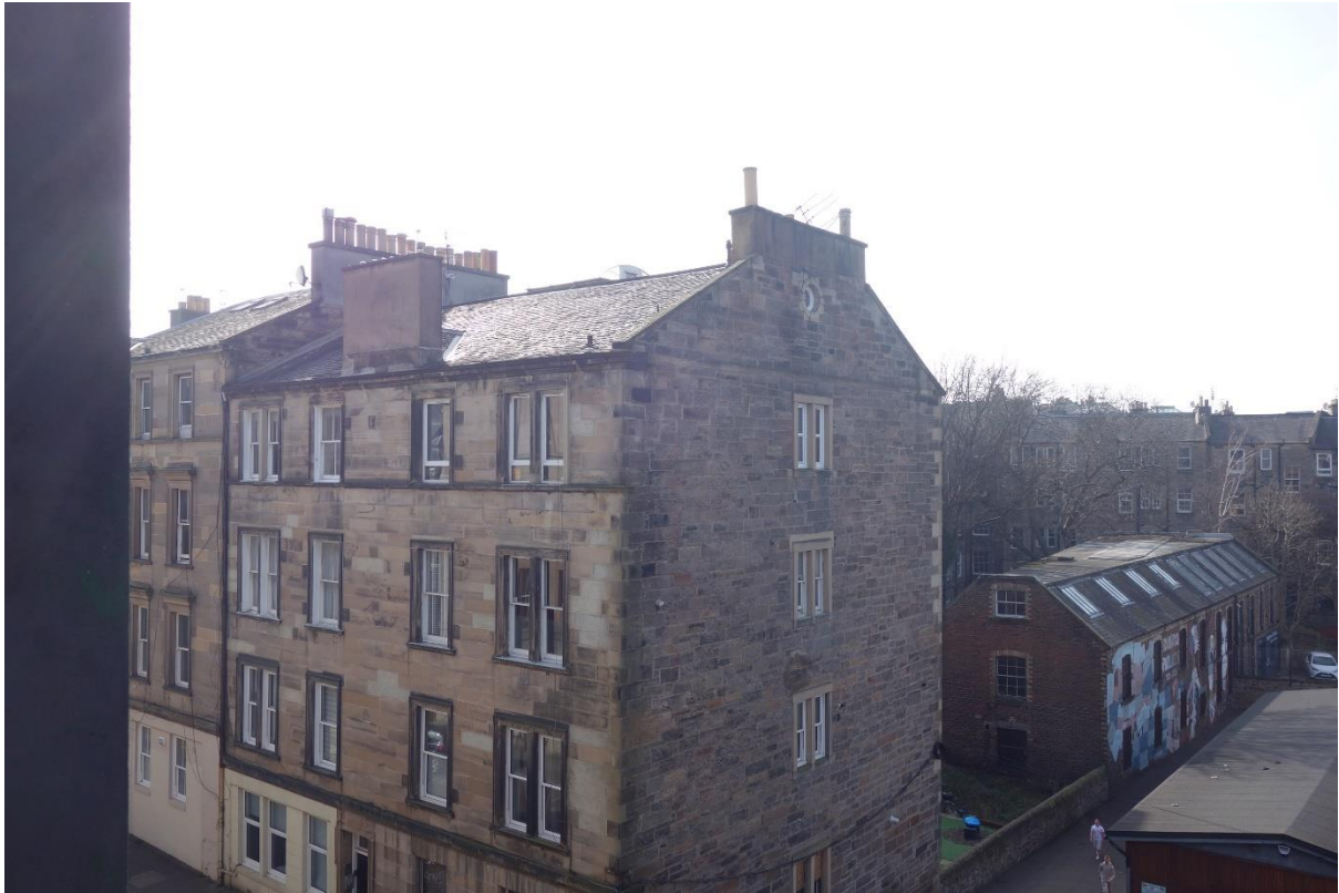
West Montgomery Place viewed from 3F1
