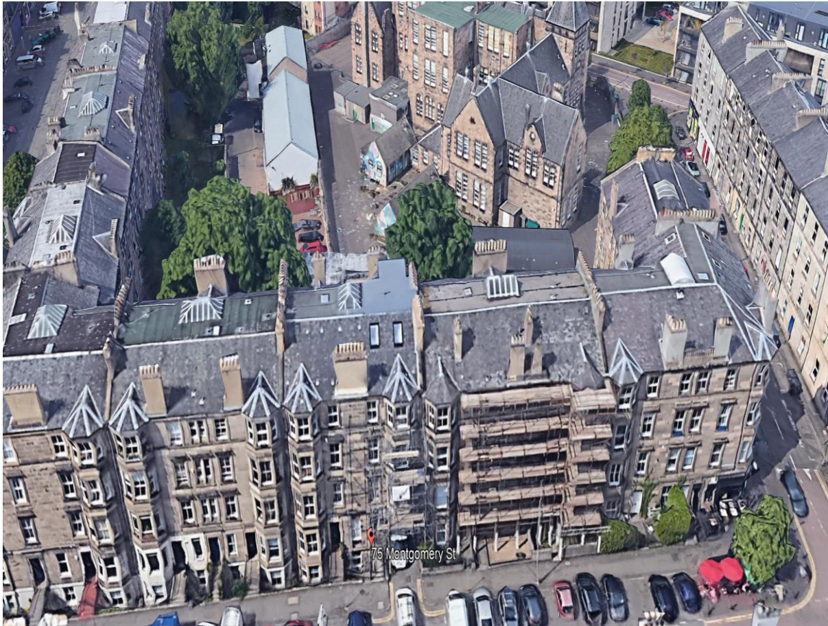
Figure 2 Planning permission for a similar scheme was granted at 75 Montgomery Street which is in a Conservation Area
