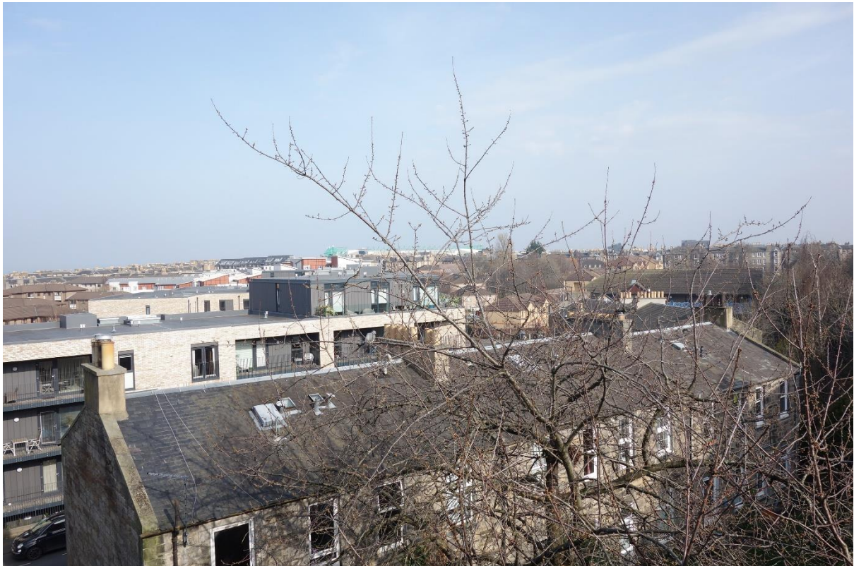
The adjacent modern apartments interestingly include roof extensions in their design philosophy, which would be compatible with the proposal.
